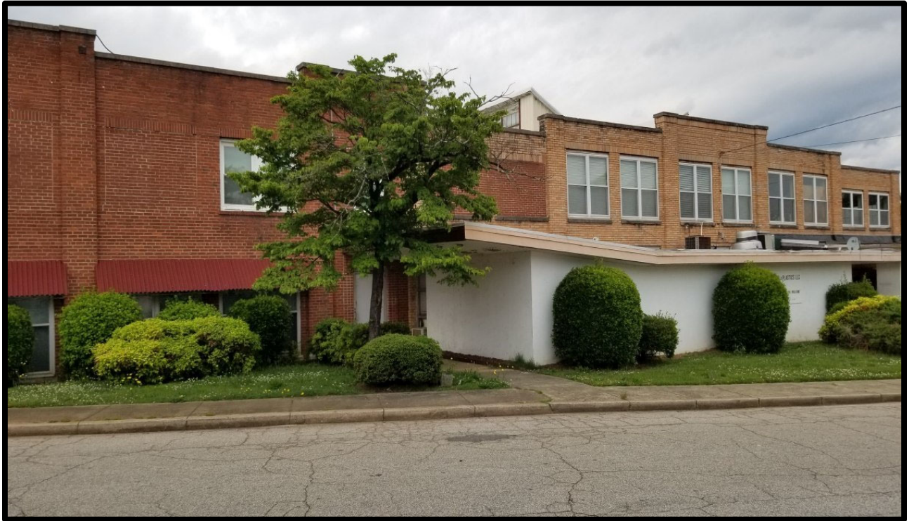
Photo 1 – existing buildings on the site
